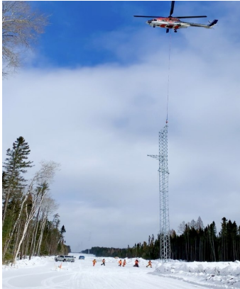
Setting the final Tower
