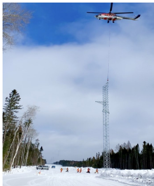
Setting the final Tower
