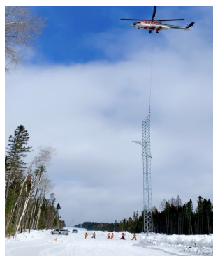
Setting the final Tower
