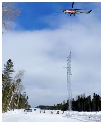
Setting the final Tower
