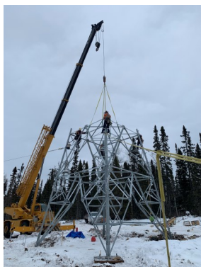
PQ Section Conventional Crane Erection
