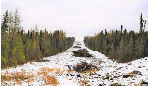
Cleared Right of Way North G1
