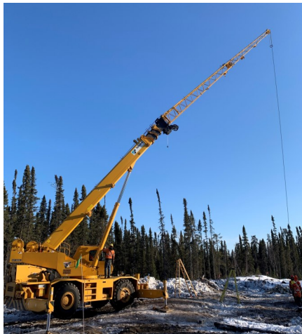
Conventional Tower Erection North G1
