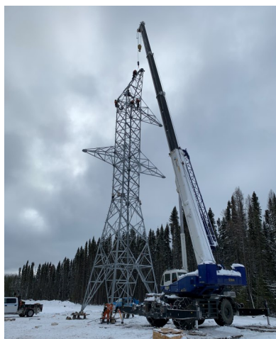
Conventional Tower Erection North G1
